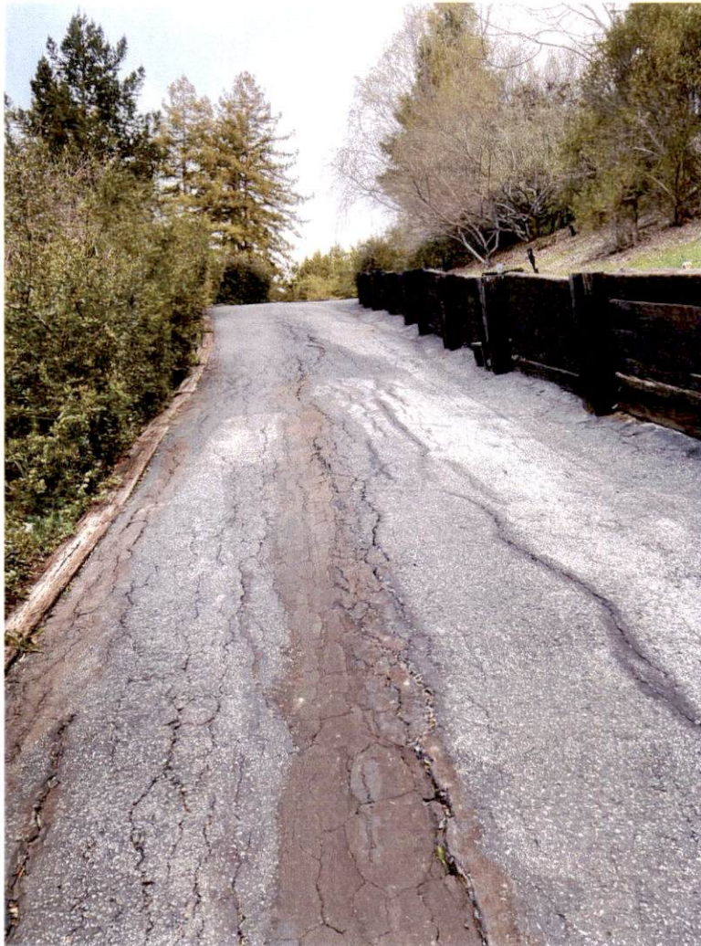
Photo 2 — Looking north and upslope the entrance at 10707 La Honda Road, Woodside, CA 94062 (San Mateo County) (Assessor's Parcel 078-190-210), the wood retaining wall (right side of photo) will be replaced after the driveway is widened as part of the Project.
