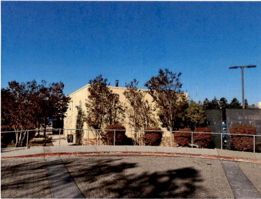
Photograph 3: Glenn Kovas Aquatic Center, camera facing northwest, December 3, 2024.
