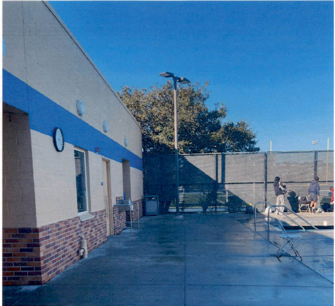
Figure 3 – Existing Light Poles (Aquatic Center)
