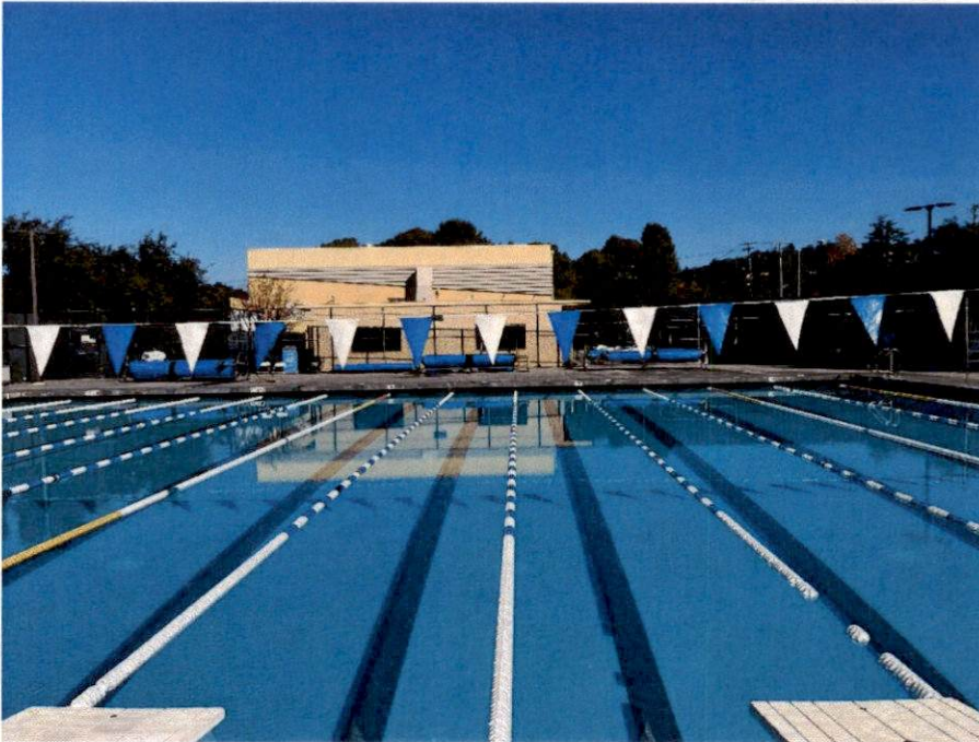
Photograph 4: Glenn Kovas Aquatic Center, Scot's Gym background, camera facing northeast, December 3, 2024.
