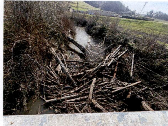
Photo 1. Pescadero Creek Bridge, facing upstream (2/18/2025).
